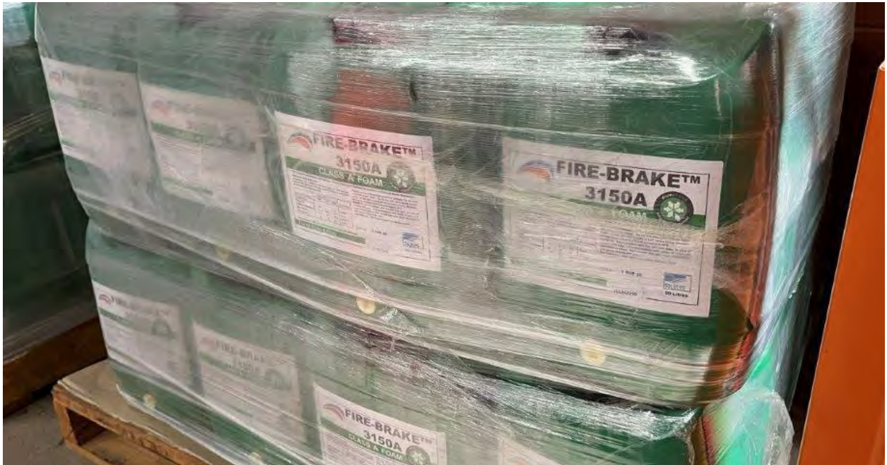
Photo 8 Current (2022) foam storage, held within the 'No. 2 Engine Room' on pallets'
