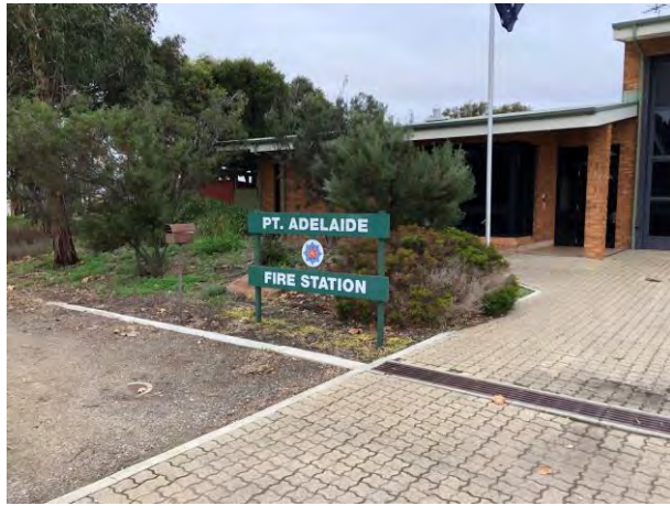
Photo 1 View of Entrance, facing S, from Grand Junction Rd
