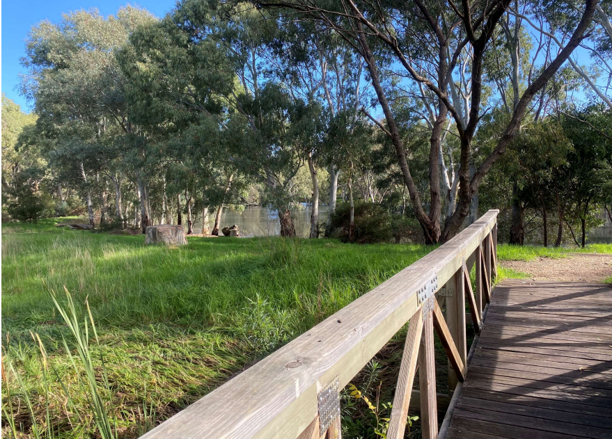
Photo 1 Bridge access within Park 23 (Wirranendi).
