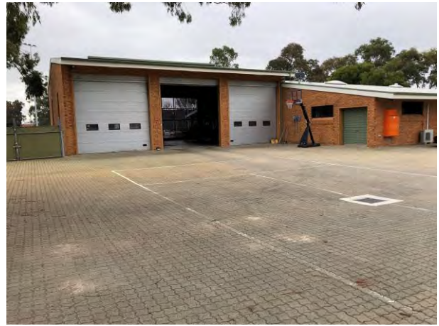
Photo 38 Rear recreation area and washdown bay, facing north
