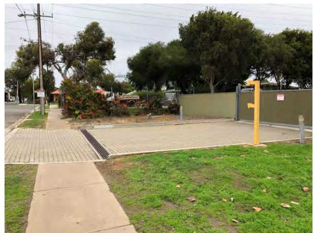
Photo 42 View vehicle access and drain from Langham Pl, facing W
