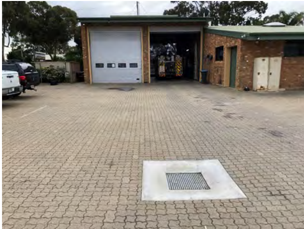
Photo 7 Rear yard training and wash down area facing north towards the engine bay and Grand Jct Rd
