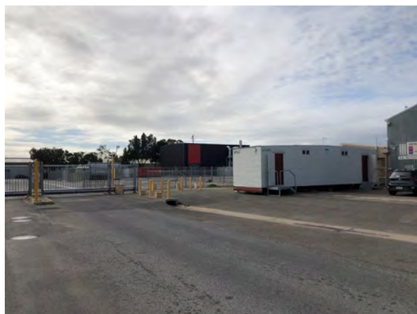
Photo 3 Gutter draining north towards Grand Jct Rd with former location of high-expansion foam training building in background, facing north-east
