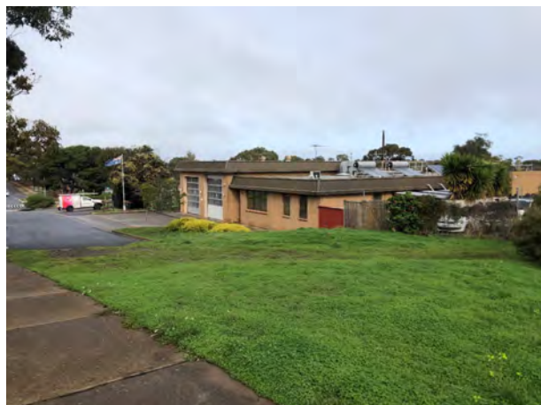
Photo 1 View of station from the north-east corner of the site
