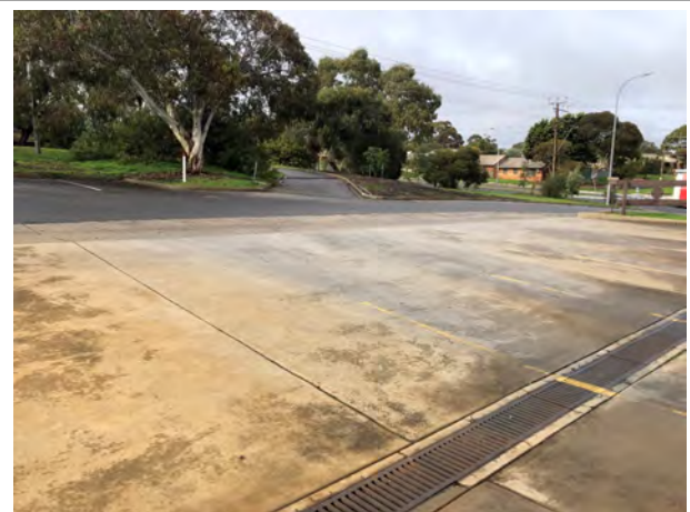
Photo 12 Wash down area in front of the station facing south-east towards the Holman Rd / Flaxmill Rd
