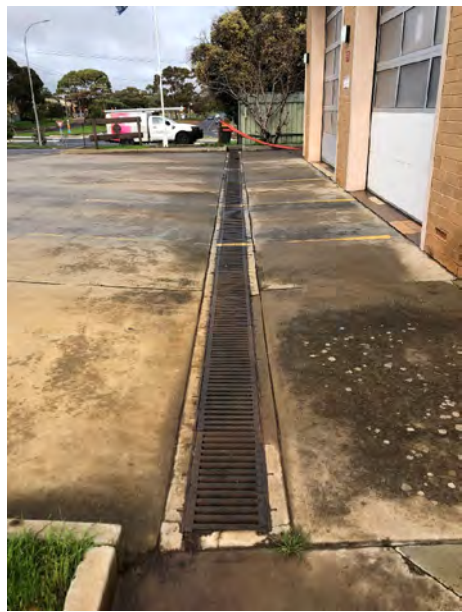
Photo 8 View of stormwater drain, facing south towards Flaxmill Rd
