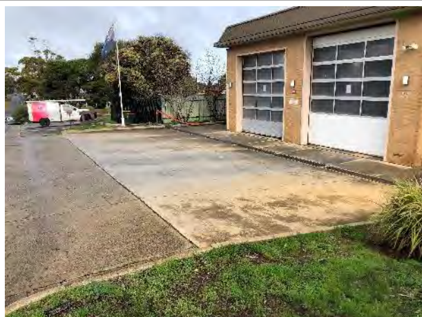
Photo 3 View of engine bay and wash down area with drain, facing south-south-west
