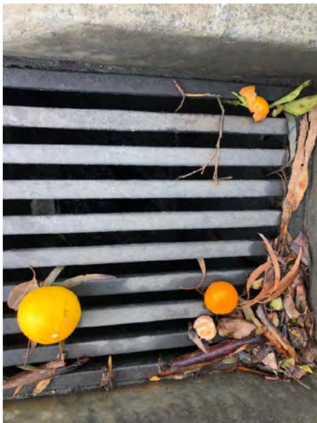
Photo 9 Close up of stormwater drain
