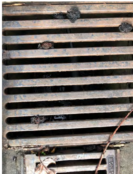
Photo 10 Close up of stormwater drain
