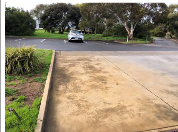
Photo 11 Wash down area in front of the station with the carpark on Holman Rd beyond, facing east
